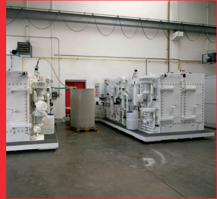
Sewage Treatment Systems
